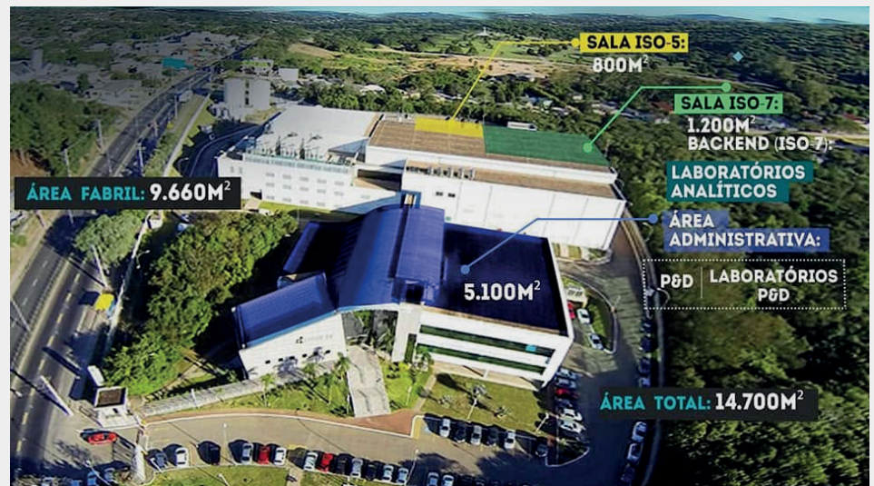
CEITEC's semiconductor complex in Porto Alegre spans 14,700 m², including 9,660 m² of manufacturing space, dedicated R&D and analytical laboratories and ISO-5 and ISO-7 cleanrooms. CEITEC has produced more than 245 million semiconductor devices over its history, giving the company an established industrial base and substantial manufacturing experience. This infrastructure is one of the reasons CEITEC can play a central role in Brazil's effort to expand semiconductor manufacturing and advanced SiC capabilities domestically. (Source: CEITEC )
